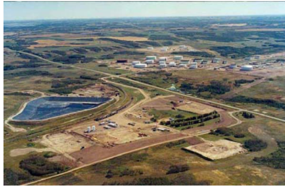
Figure 1: Aerial view of Cavern site and Hardisty Oil Hub
